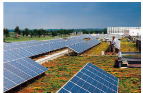
6. Roof with fully-installed solar energy system.
