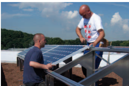
5. The solar panels are installed.
