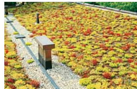
This roof with a pitch of approx. 5° is drained using a gutter and does not yet require any special measures.
