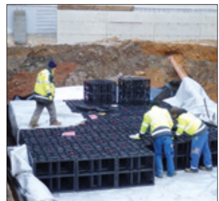
Industrial building, Tumeltsham (AT)
