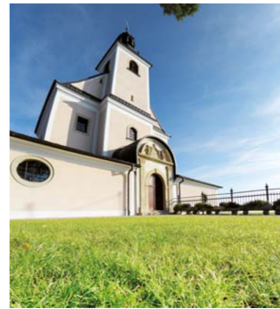
Green fire escape route, Sanctuary in Bystrzyca Kłodzka
