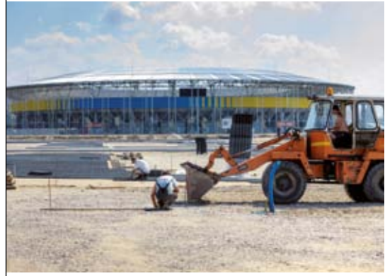
load bearing layer distribution
