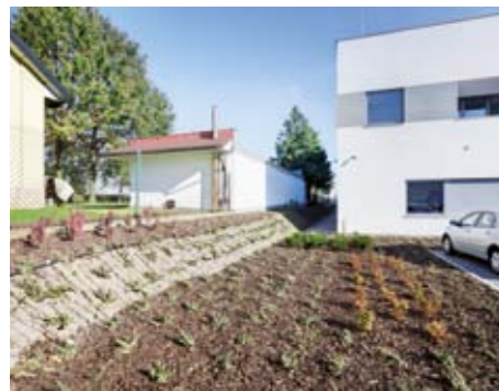
Slope reinforcement, Warsaw
