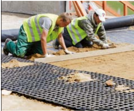
distribution of the leveling layer
