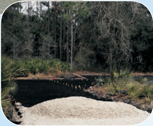
Preparing the base by placing a geotextile fabric over the muck soil. Next, Geoweb sections were placed over the geotextile fabric, staked and infilled with #57 stone.
