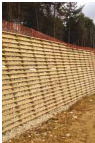
Center Parcs, Woburn, Timber Crib
