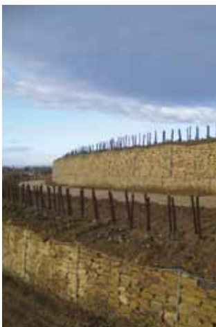
Rotherham Cemetery, Gabions
