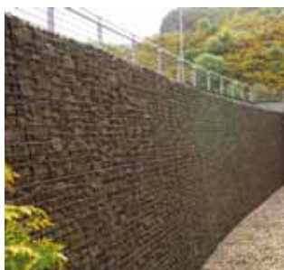
Napier University, Edinburgh Gabions
