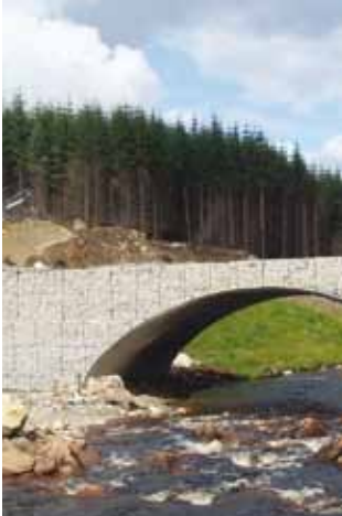
Wind Farm, Inverary, Gabion Terramesh®
