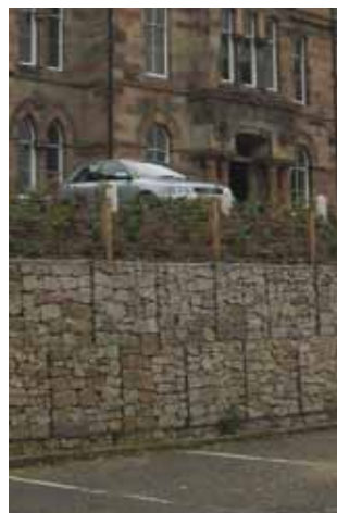
Langside College, Glasgow, Gabions
