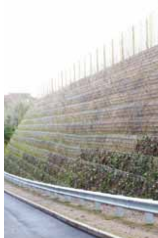
Duncans Road, Lisburn, Green Terramesh®
