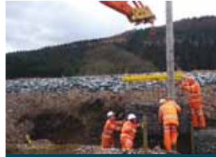
Dalguise, Perthshire, Installation of Prefilled Gabions
