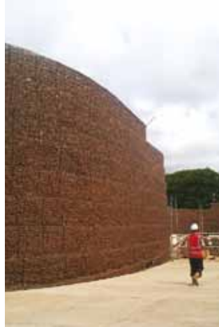
Glencorse Water Treatment Works, Gabion Terramesh®
