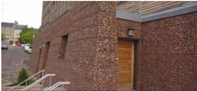
Edinburgh University, Gabion cladding
