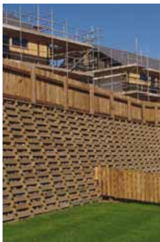
Lochside, Dumfries, Timber Crib
