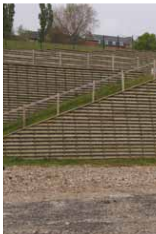
Loadman Street, Newcastle, Timber Crib
