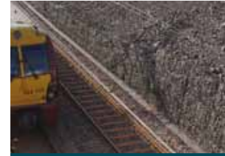
Airdrie Bathgate Rail Line, Airdrie, Installed Prefilled Gabions
