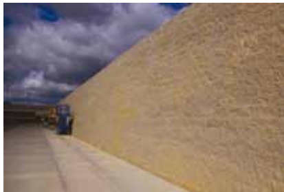
BMW Cowley, MacWall™
