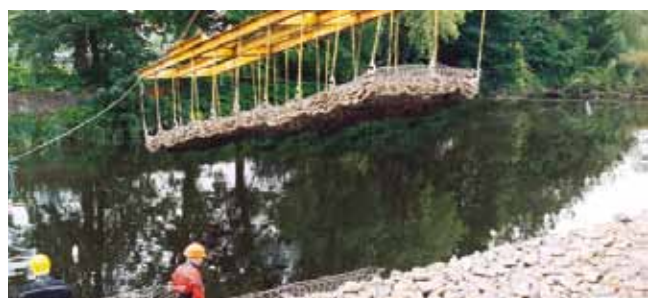
Anchor Mills, Paisley, Erosion Protection
