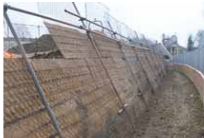
Hackbridge, London, Green Terramesh®
