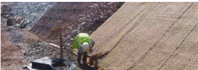
A90, Portlethan during construction Aberdeen, GeoMac®
