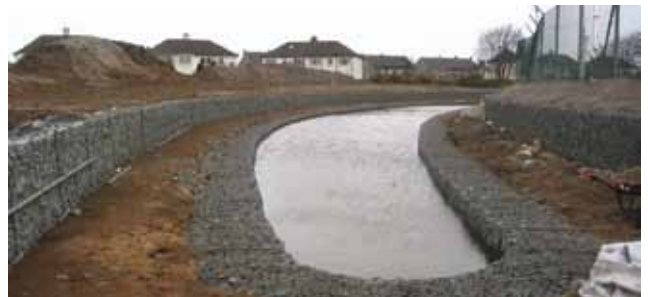
Prestwick during construction, SUDS
