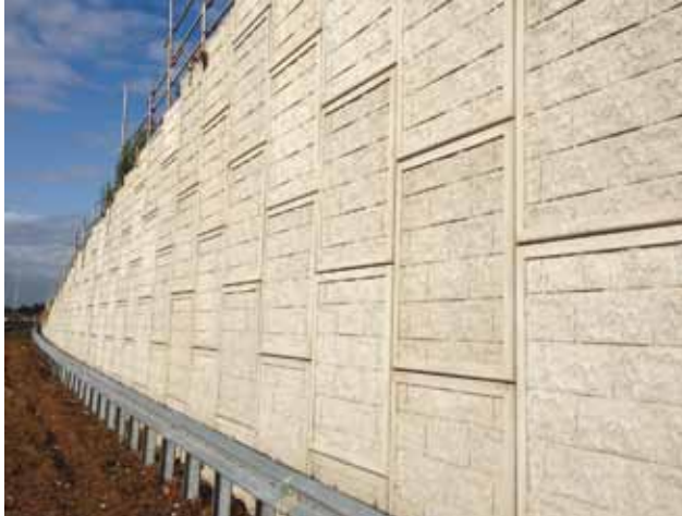
Sadlers Farm junction improvements, MacRes®
