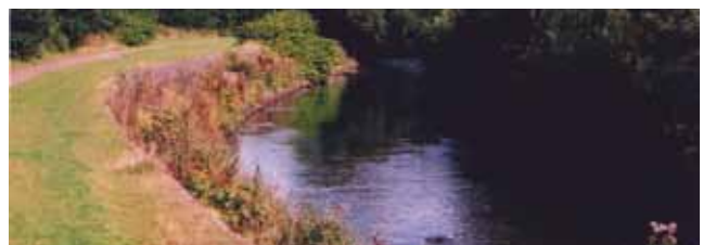
Inveresk, Midlothian, Erosion Protection, post construction
