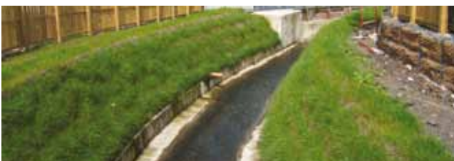
Saucel Street, Paisley, Erosion Protection, post construction
