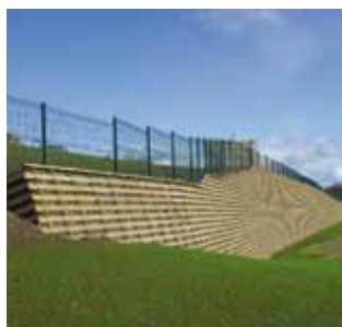
Loadman Street, Newcastle Timber Crib
