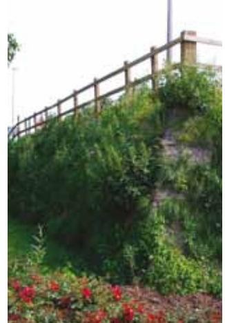
A5130 Improvements, Milton Keynes, Green Terramesh®
