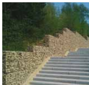
Langtrees, Liverpool, Gabions
