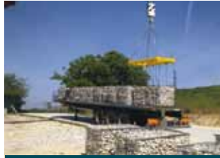
DIRFT, Daventry, Loading of Prefilled Gabions
