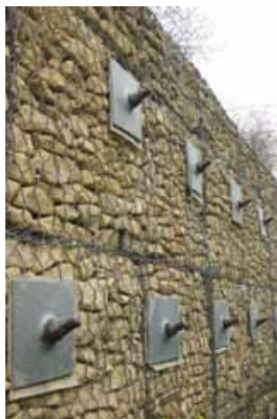
Northolt Embankment, Ruislip, Gabions
