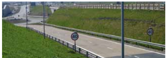
A90, Portlethan post construction, Aberdeen, GeoMac®
