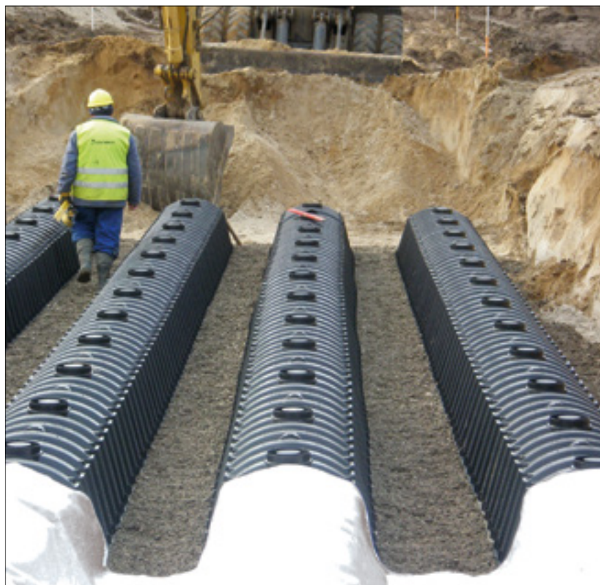
Industrial warehouse, Raben (PL)
