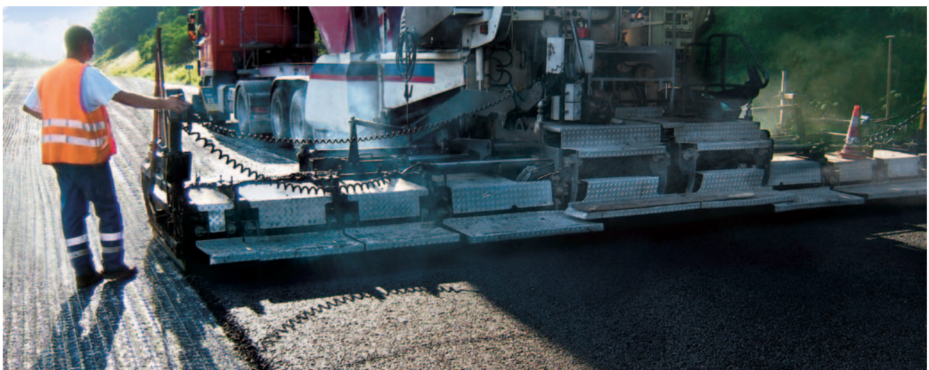
Paving takes place directly over the Tensor AR-GN.
