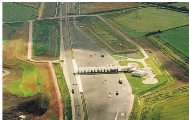
Second Severn Crossing Bridge Toll Plaza supported on Tensar geogrid LTP (UK).
