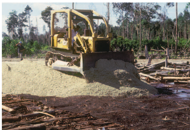
Road construction using an LTP over peat (Indonesia).
