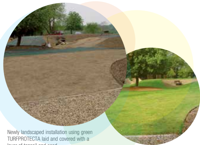
After just a few weeks the grass grows through the mesh offering a strong stabilised surface.
