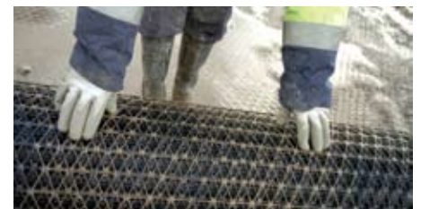
TriAx geogrid unrolled on site.
