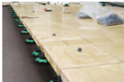
Elefeet® H 50 adjustable from 52 up to 82 mm
