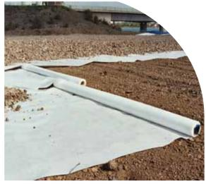
Permeable filter/separator geotextile for separating sub-base construction layers from intermixing.
