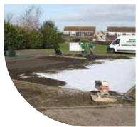
Terram non-woven standard geotextiles deliver separation and filtration. They are resistant to all naturally occurring soil acids and alkalis and is unaffected by biological contaminants such as bacteria or fungi.
